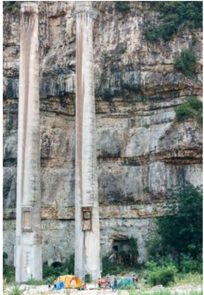
Occupy the ex Italcementi factory. © WK
