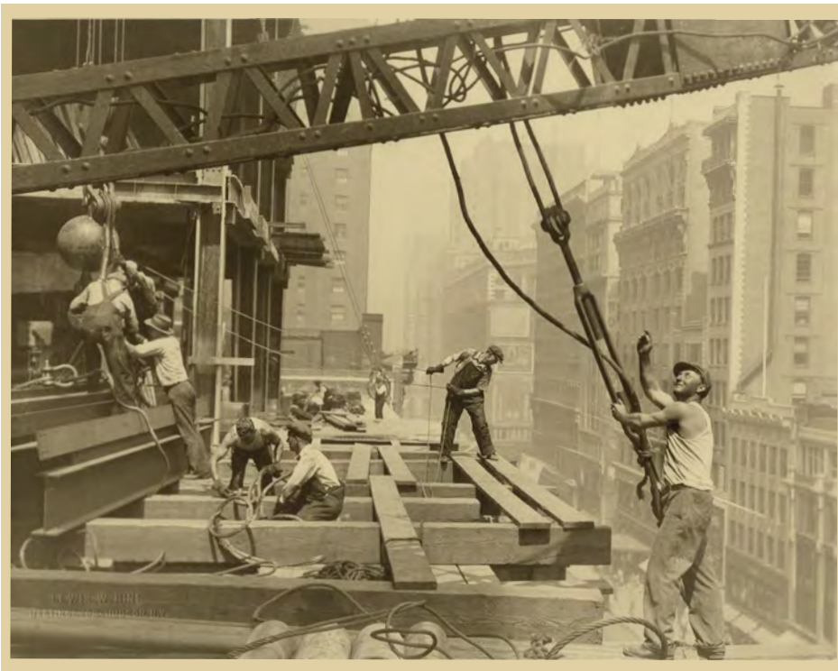
Fig. 7. Lewis Wickes Hine, Empire State Building Construction (1930). Permanent Loan to MCNY.
